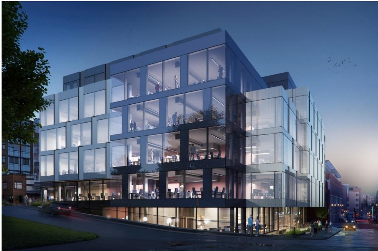
Gullhaugs Torg 5 in Oslo, Norway
